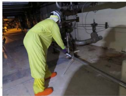
Installation of ultrasonic transducer and clamp
