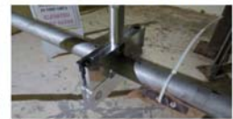
Installed ultrasonic transducer and clamp
